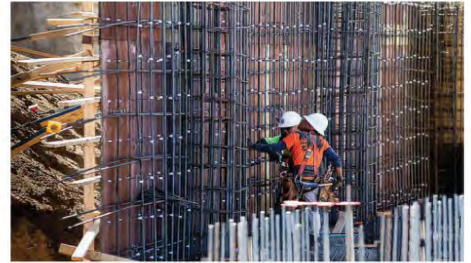
Above & Below: Rebar serves as a tension device in the reinforced concrete that Alliance Construction is self-performing.
