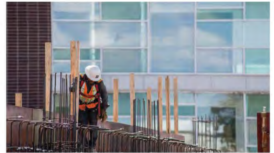
Above & Below: Rebar serves as a tension device in the reinforced concrete that Alliance Construction is self-performing.
