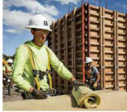
Foundation walls are currently going in on The Source Hotel site.
