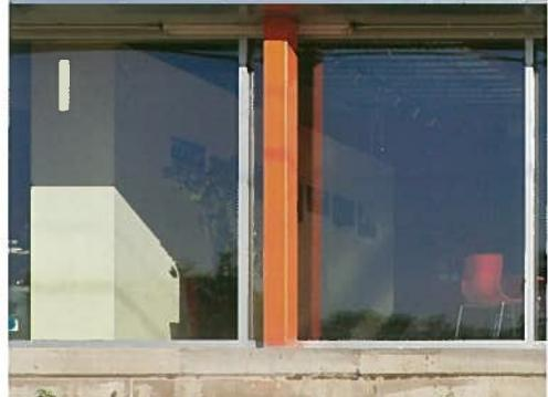
The former goods terminal contained a main building with one floor with a face brick finish. Reusing the facade involved replacing the original factory brick with a much lighter brick. Metal elements were used, along with fixed glass windows. An intermediate framework was built and the roof level was raised.
