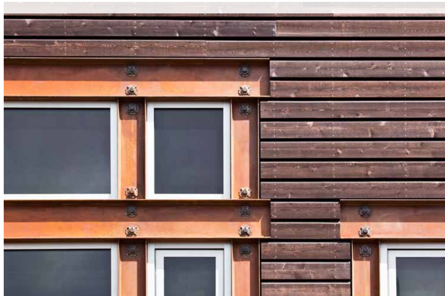
THIS PAGE, UPPER Finishes change the character of steel cladding, as exemplified by this oxidized treatment by Teton Heritage Builders. PHOTO Courtesy of Teton Heritage Builders. THIS PAGE, LOWER A mix of wood slats and riveted oxidized steel reflect a daring design ethos. PHOTO Courtesy of Atelier One Ltd. OPPOSITE Teton Heritage Builders is pleased with the performance of steel cladding, so much so, they clad their own office. PHOTO Courtesy of Teton Heritage Builders.
